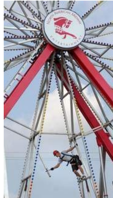
A worker with North American Midway Entertainment helps construct a ferris wheel at the Mississippi Fairgrounds in Jackson on Tuesday in preparation for the State Fair, which kicks off today. (Joe Ellis/The Clarion-Ledger)
